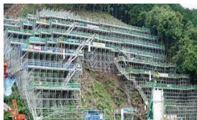
YT Lock System enables assembly of platforms for cranes and other heavy equipment without any tools
