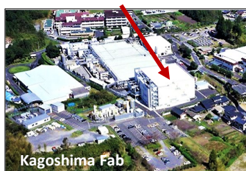
Annex for new clean room
