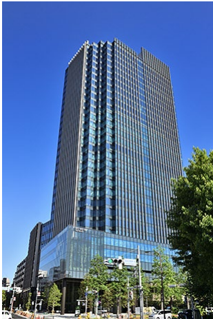
Head Office Building (1-6-1, Shinjyuku Yotsuya, Tokyo)
